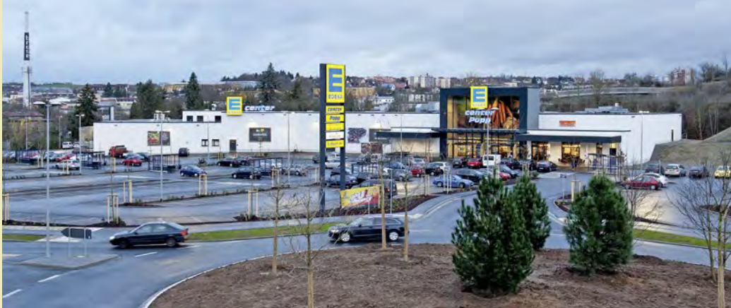
Schlüsselfertiger Neubau des Edeka-Center Popp in Würzburg (Foto: Katrin Heyer)
